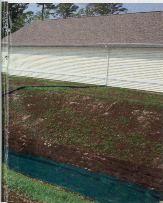
Top, left to right: McGill Premium Compost used a blower truck to compost and reseed a range field at Camp Lejeune, NC. Above, left to right: A stream bank restoration at Camp Lejeune leading to a retention pond. The project used erosion control socks with McGill SoilBuilder Premium Compost.
