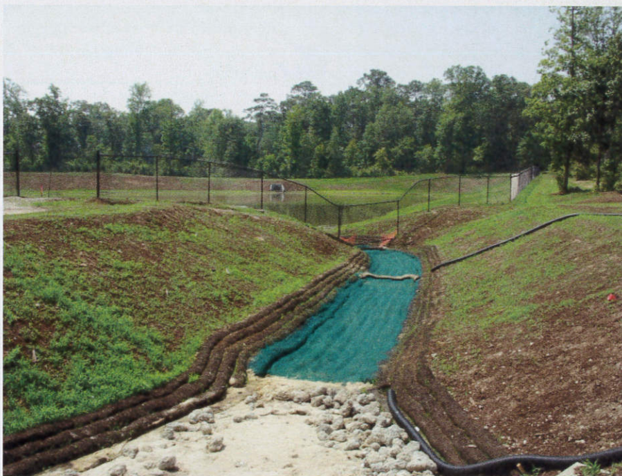
Top, left to right: McGill Premium Compost used a blower truck to compost and reseed a range field at Camp Lejeune, NC. Above, left to right: A stream bank restoration at Camp Lejeune leading to a retention pond. The project used erosion control socks with McGill SoilBuilder Premium Compost.
